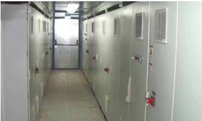
Power panels within the “Powertainer”
