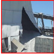
SILO RUPTURE
